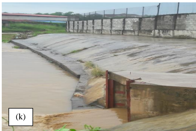
Figures 5.6: (k) and (l) Reinforced concrete embankment and wall fence constructed to prevent flooding at Yale Foods Limited, and Rhema Chapel respectively at Oluyole Industrial Estate, Oluyole LGA
