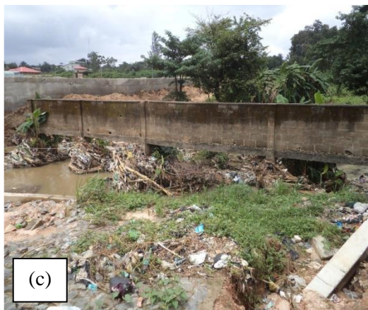
Figures 5.3: (c) Drainage channel and hydraulic structure blocked by solid waste along the University of Ibadan wall fence (d) Solid waste dumped on Mokola stream, Mokola area
